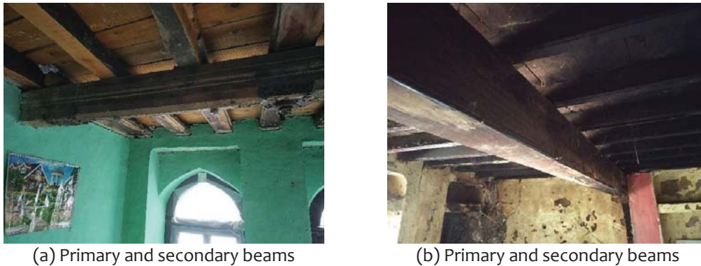
Figure 2.59: Floor system in Dhajji-Dewari buildings
