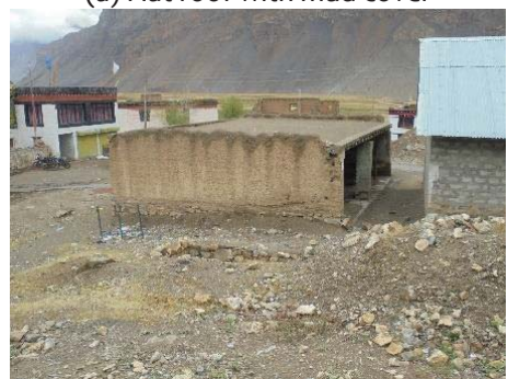
(c) Flat roof with mud cover
