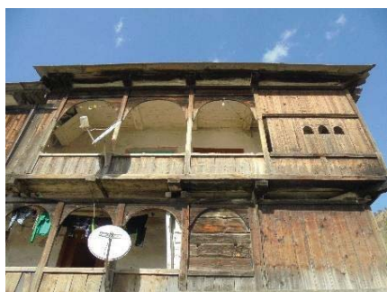
(a) The gap between adjacent buildings
