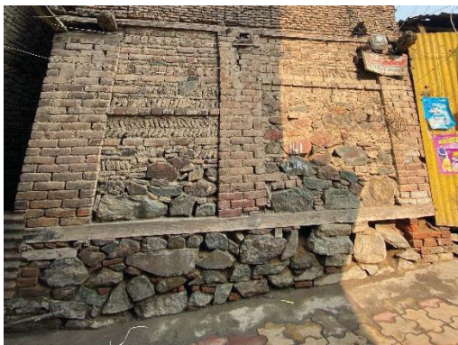
(a) Stone foundation
