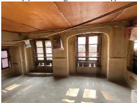
(c) Internal view of Taq piers
