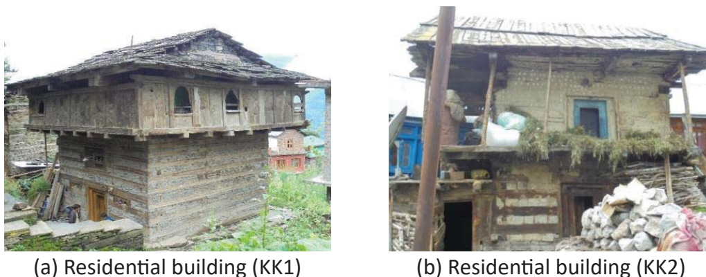
Figure 2.4: Variants of the Kath-kunni buildings observed in the study region
