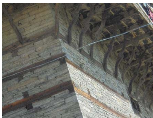
(b) Wall thickness @ 0.90 m
