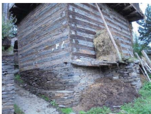
(c) On a raised dry-stone platform
