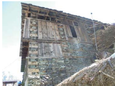
(b) Wall thickness @0.45m
