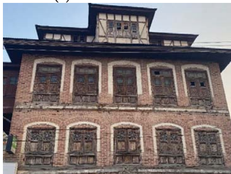
(c) Openings between Taq piers
