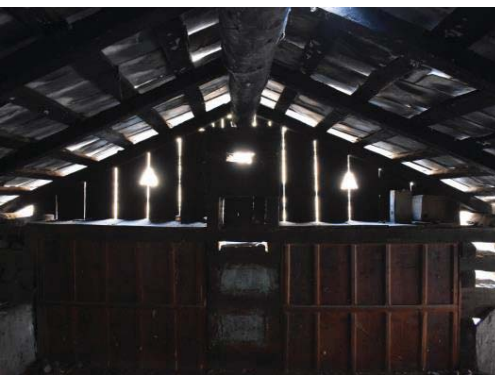
(c) Nhas with rafters spaced @ 1.2 m
