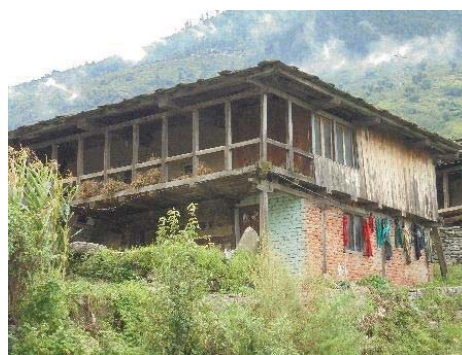
(b) Brick walls in Kath-kunni
