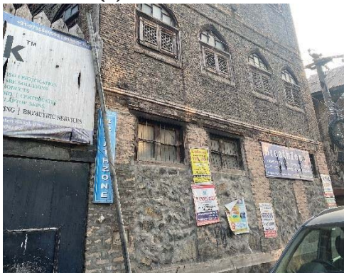
(c) Plinth band on the stone foundation
