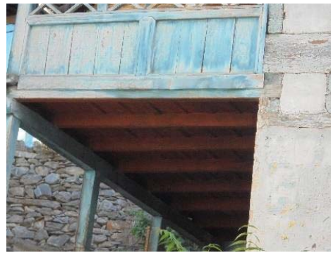
(b) Primary and secondary floor beams
