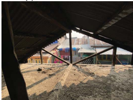
(c) Roof system
