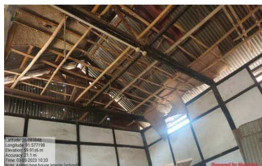
(e) King post truss with braces
