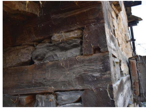
(b) Wall-to-wall connections
