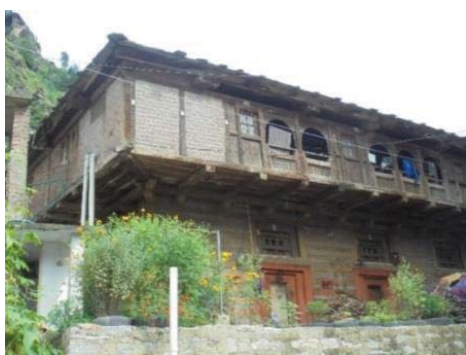
(a) Brick walls in Kath-kunni
