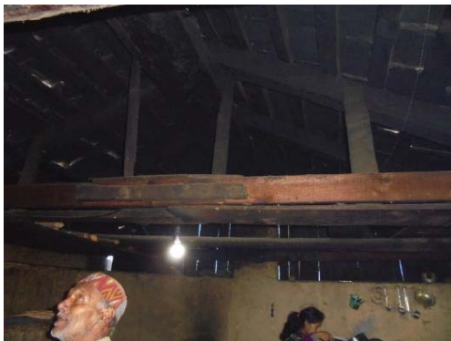
(a) Trussed roof system
