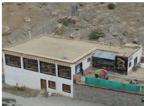
(a) Flat roof with mud cover
