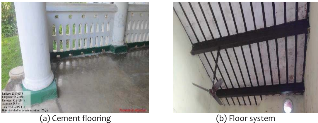
Figure 2.103: Floor system in Assam-type buildings
