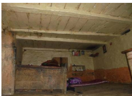
(c) Timber planks on timber floor joists
