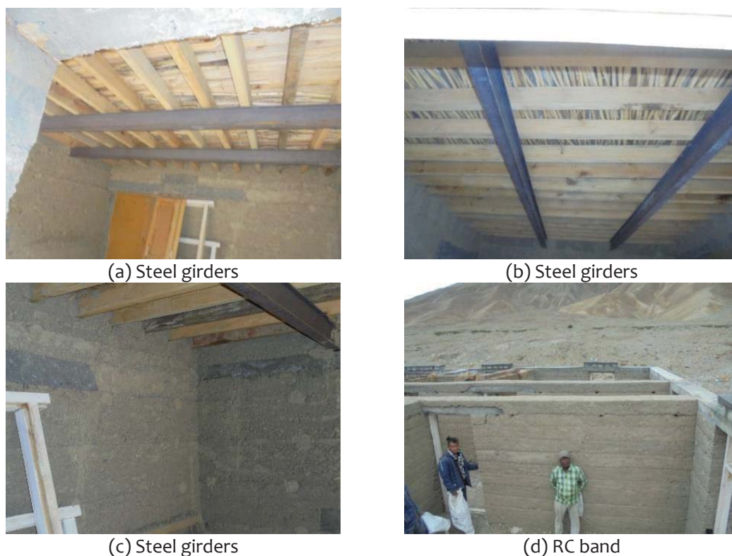
Figure 3.18: Influence of contemporary materials in rammed earth buildings
