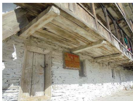
(b) The gap between adjacent buildings
