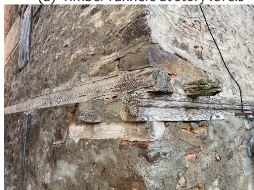
(c) Timber runners with cross-piece
