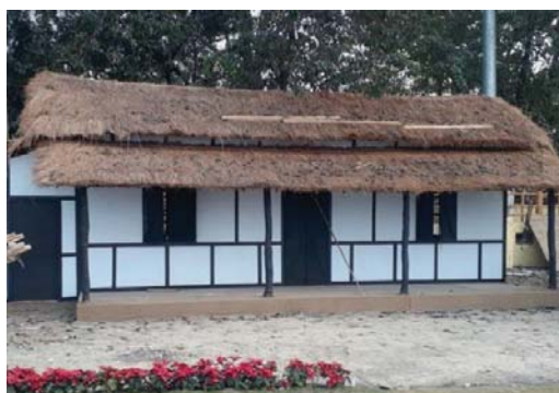
(a) Gable roof with Thatch
