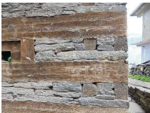
(a) Wall thickness @ 0.30 m
