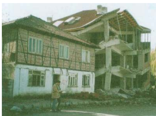
(a) Duzce earthquake, 1999 (Langenbach 2020)
