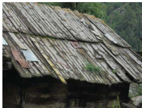
(b) Gable roof with timber planks
