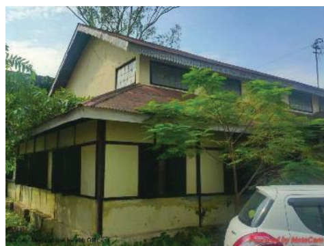
(b) Closely spaced openings
