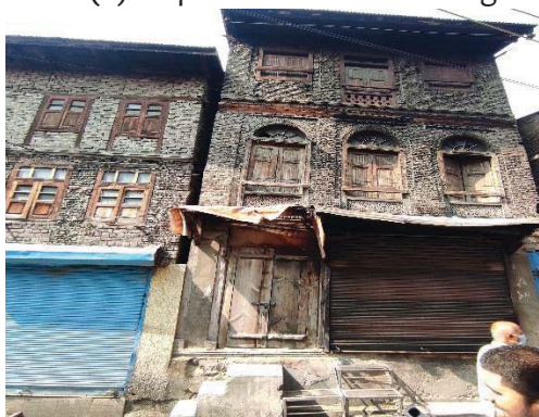
(c) Gap between two buildings
