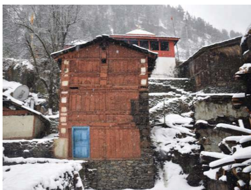
(e) On raised dry-stone platform
