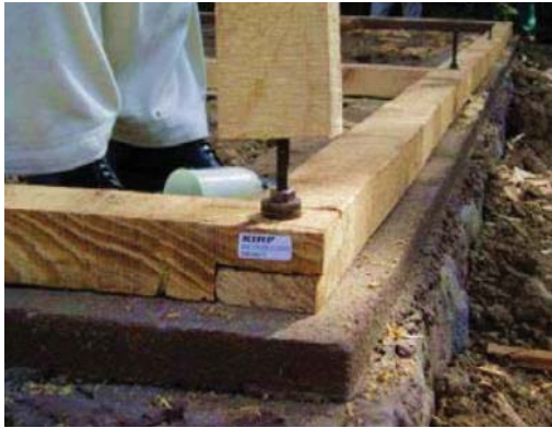
(a) Bolting of plinth beam to foundation
