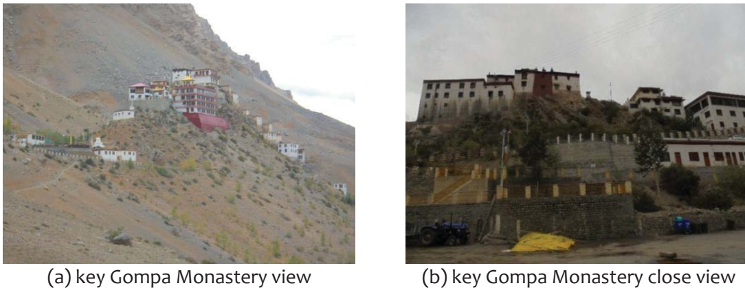
Figure 3.2: Rammed earth buildings on hill slopes in Spiti Valley – Key Gopa Monastery
