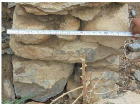
(a) 0.45m thick stone foundation
