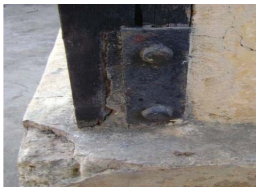
(b) Post-bolted to foundation
