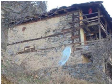
(c) Thola-to-wall connections
