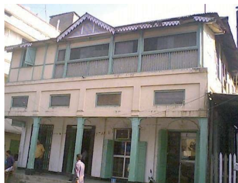
(b) Timber frame and bricks
