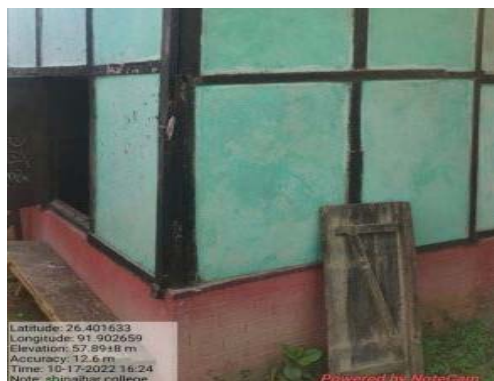
(a) Masonry foundation
