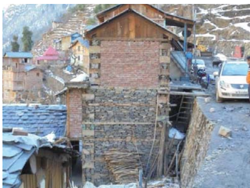
(a) Burnt clay brick walls
