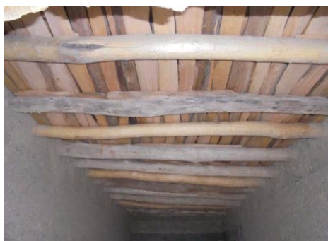
(a) Bamboo and split timber elements
