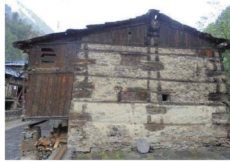
(b) Floor beam in Thathara buildings
