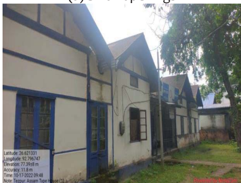
(c) Uniformly distributed large openings
