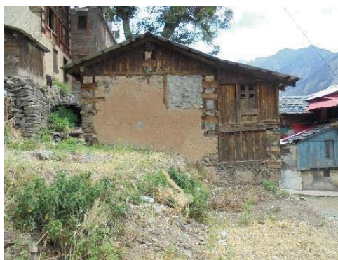
(b) Two foundation level
