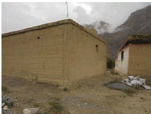
(a) Gap between buildings
