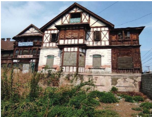
(a) Hospital building
