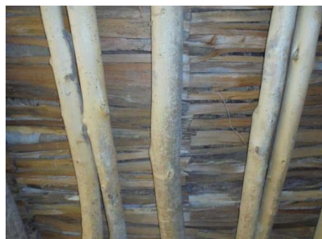
(b) Bamboo and split timber elements
