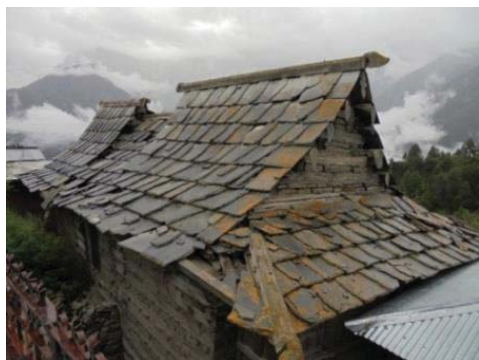
(a) Dutch-gable roof with stone slates
