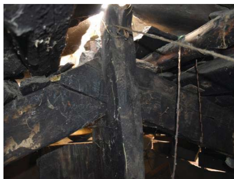
(f) Vertical posts in the roof system supporting rafters
