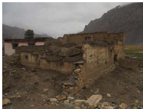
(b) Demolished building
