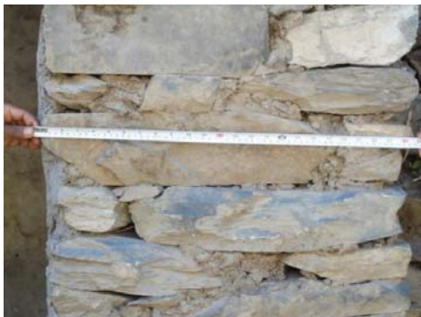
(a) Wall thickness @0.45m
