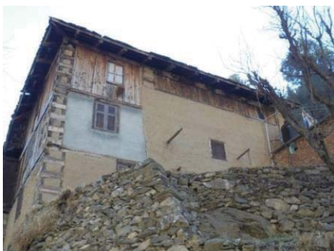
(a) Mud plaster
