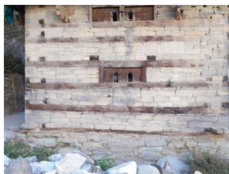
(a) Stone foundation
