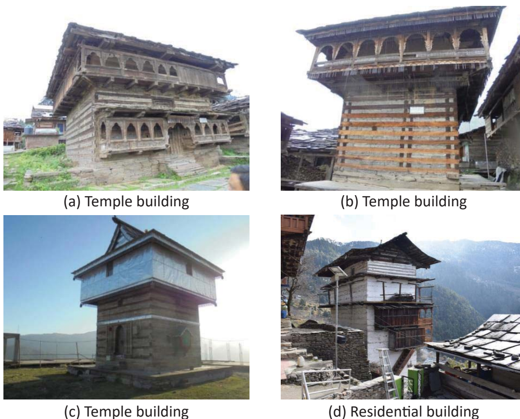
Figure 2.3: Different occupancies observed in Kath-kunni buildings
