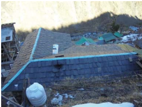
(c) Cross gable roof with stone slate
