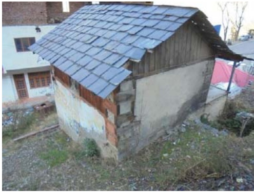
(a) Gable roof with stone slate
