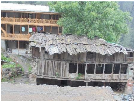
(a) Isolated building
