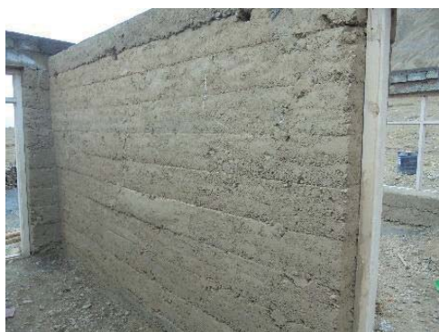
(a) Wall thickness @ 0.35 m
