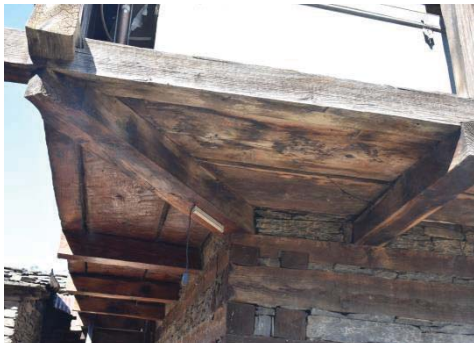
(e) Timber planks on timber floor joists
