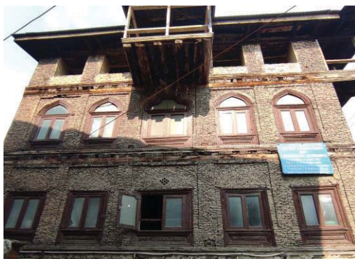
(a) Timber runners at story levels
