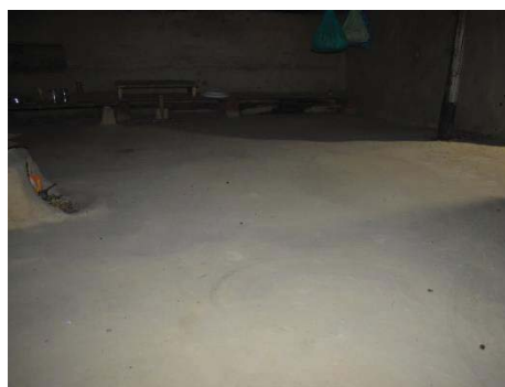
(b) Mud flooring over timber planks
