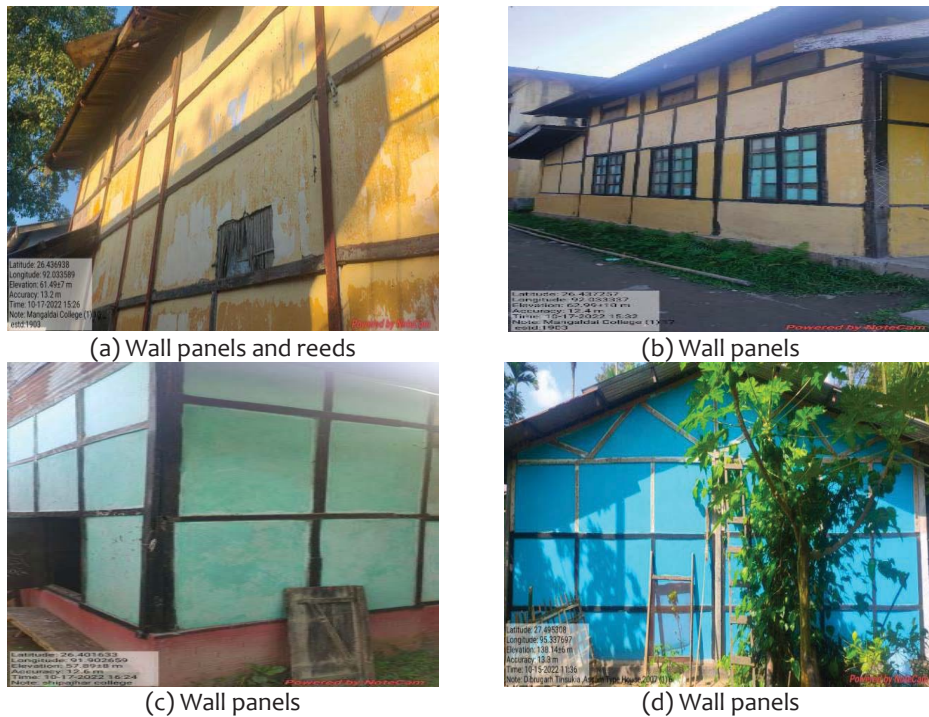
Figure 2.100: Wall system in Assam-type buildings
