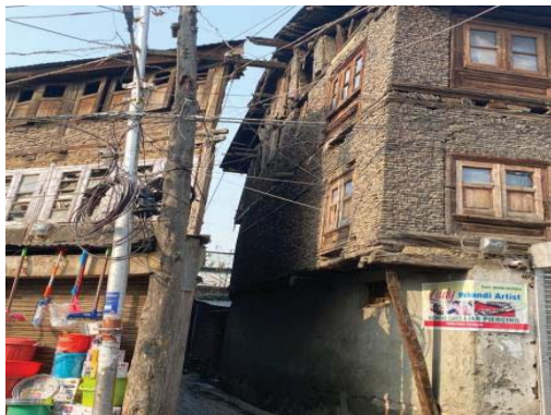
(a) Gap between two buildings
