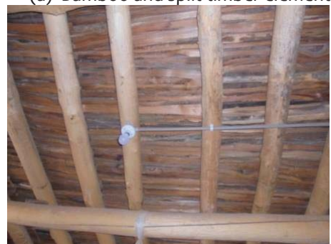
(c) Bamboo and split timber elements
