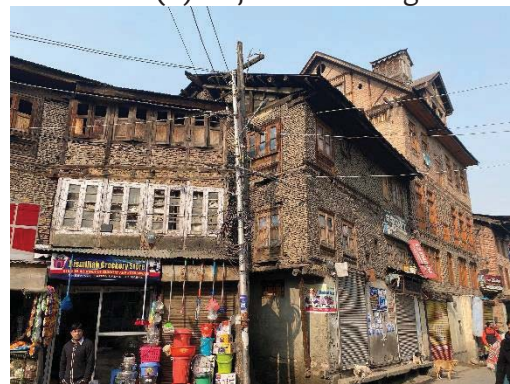
(d) Gap between two buildings
