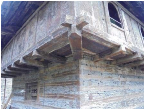
(a) Wall-to-wall connections
