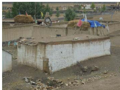
(b) Flat roof with mud cover
