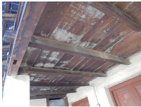
(a) Primary and secondary floor beams
