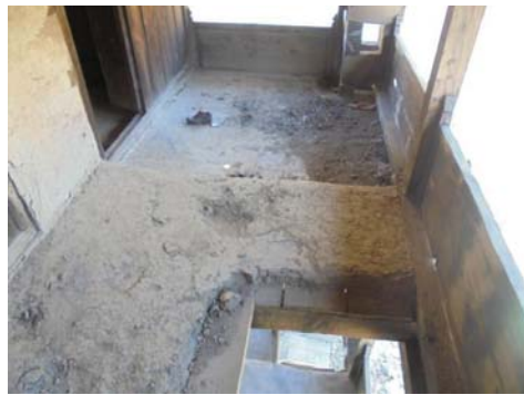
(c) Earthen cover in wooden floor
