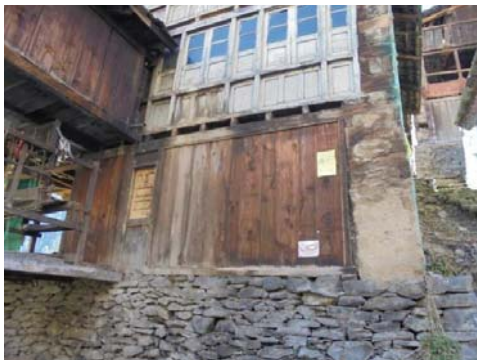
(a) Stone foundation
