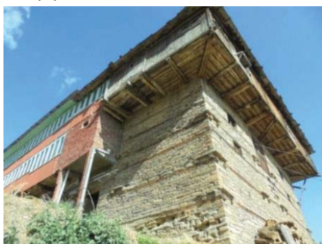
(c) Brick walls in Kath-kunni
