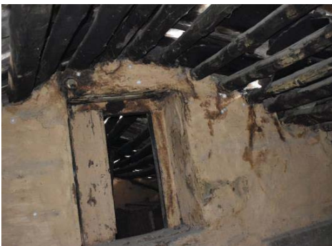
(c) Roof system
