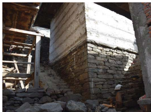
(b) On a raised dry-stone platform
