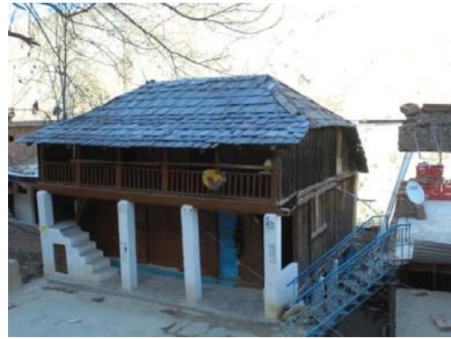
(b) Hipped roof with stone slate
