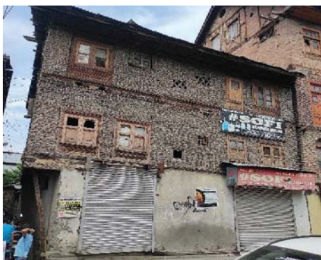
(a) Cement plaster
