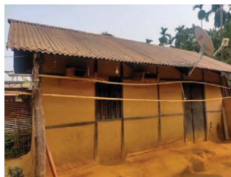
(b) Gable roof with GI sheets
