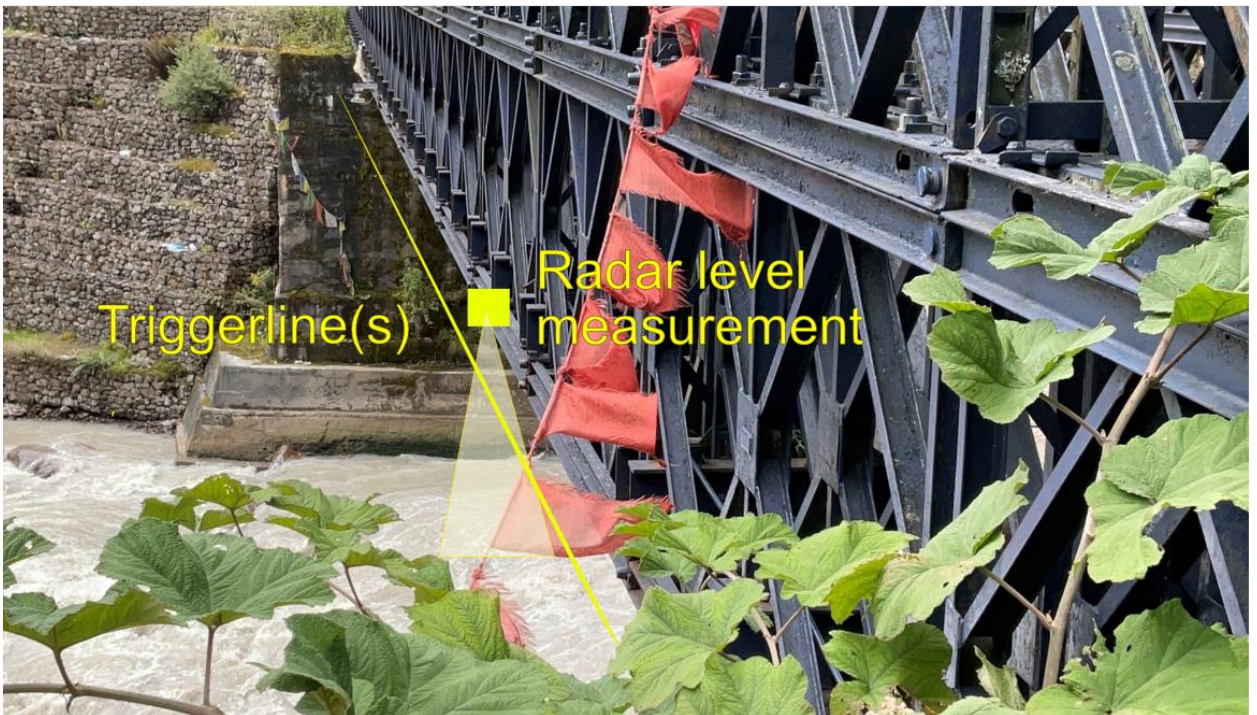
Fig. 30: Diagram showing how the trigger lines and sensors could be installed at bridge sites for generating EWS (Source: Geopraevent)
