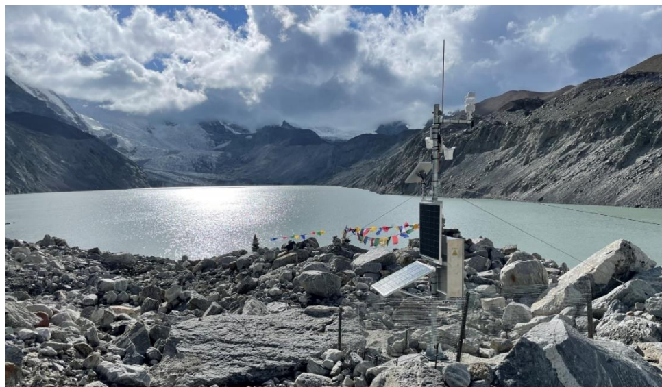
Fig. 7: Installed AWS at South Lhonak Lake (Photo clicked during the expedition)
