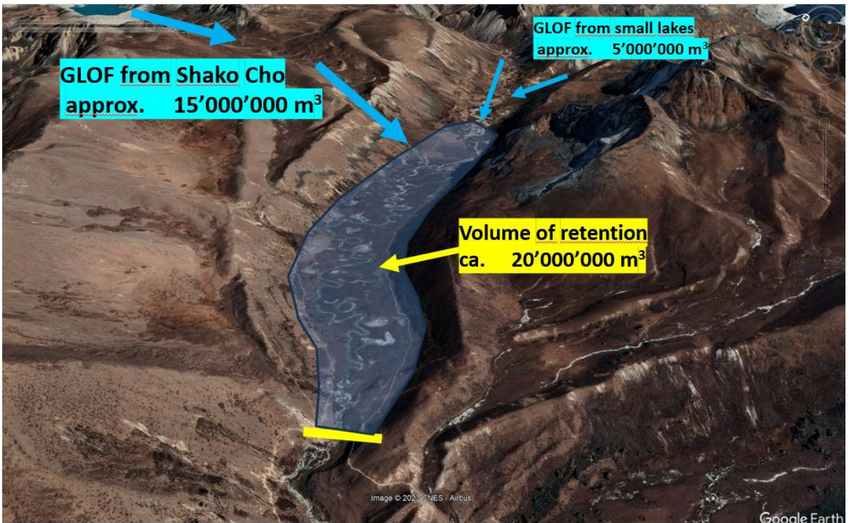
Fig. 15: Possible volume of the Retention Dam near Shako Cho Lake (Source: Geopraevent)
