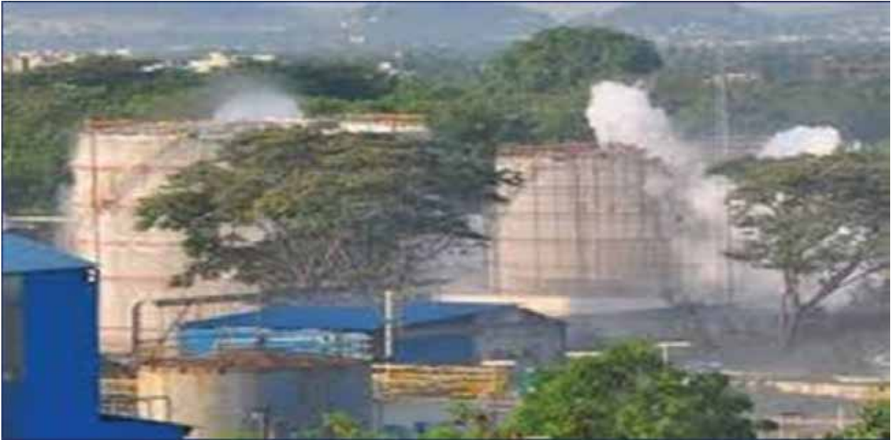
Styrene gas leak at LG Polymers Pvt. Limited, Visakhapatnam
