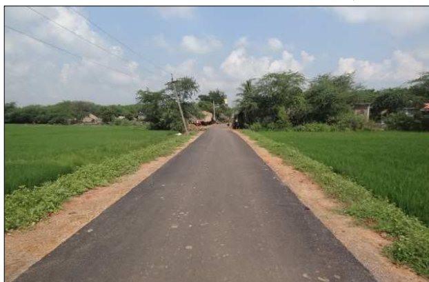
Road from R&B road to Pedagudumotu (RCH) in Krishna District (A.P.)
