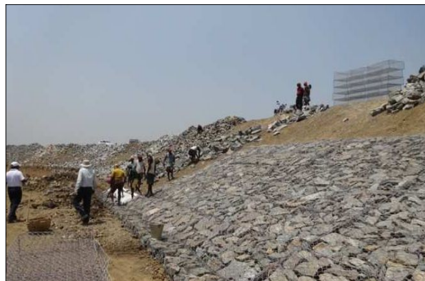
Rajnagar - Gopalpur Saline Embankment (RD. 15.05 to 19.05 Km.) Ganjam District, Odisha.
