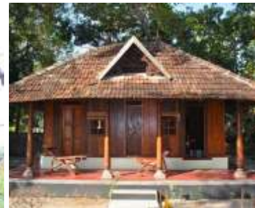
Timber walls with mangalore tiles hipped roof- Kerala
