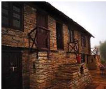
Stone rubble masonry walls with mangalore tiles gabled roof- Uttarakhand
