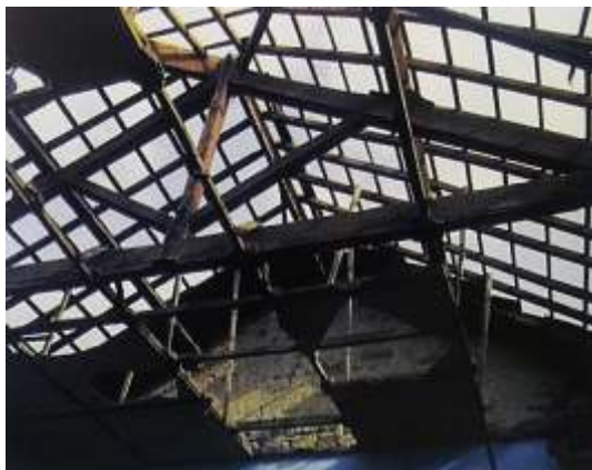
Damage to light roof due to cyclone
