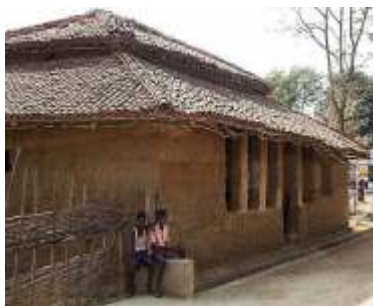
Cob walls with tiled hipped roof - Chhattisgarh
