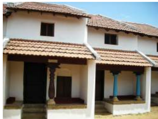
Burnt Brick walls with mangalore tiles gabled roof- Tamil Nadu
