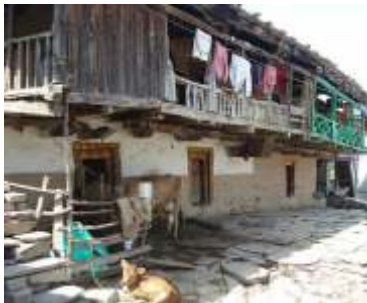
Timber walls with timber gabled roof- Uttarakhand
