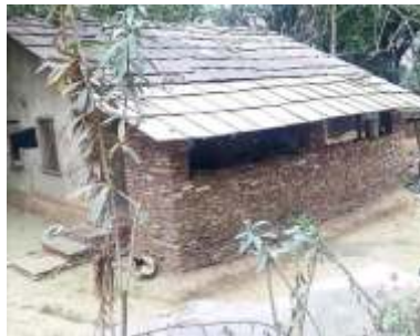
Stone rubble masonry walls with slate stone gabled roof- Chhattisgarh
