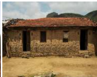
Stone rubble masonry walls with country tile flat roof- Dadra and Nagar Haveli
