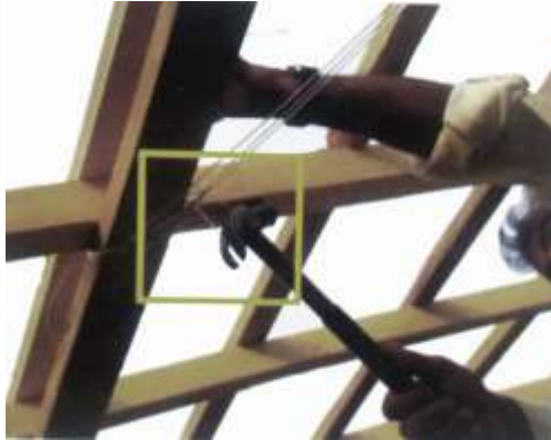
Tie one wire at a time around the joint of strut with rafter or purlin, stretched with a carpenter's hammer.
