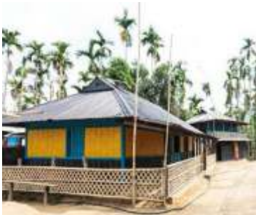
Wattle and daub walls with sheet hipped roof - Kerala
