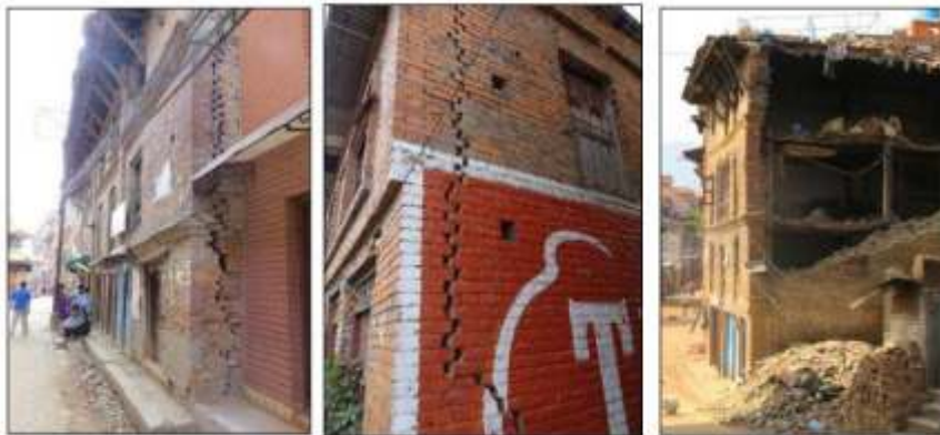
Separation of adjoining walls
