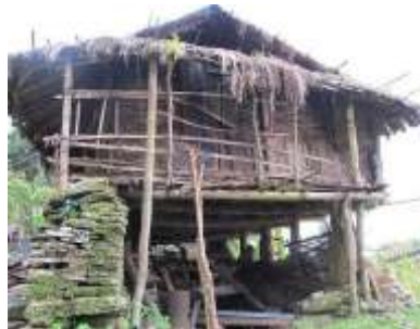
Timber walls with thatch hipped roof- Sikkim
