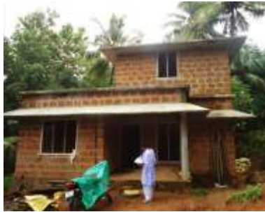
Ashlar Stone Walls with RCC flat roof- Kerala
