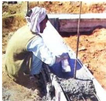
Pour concrete of 1:1.5:3 proportion with rodding. Cure band for fifteen days.
