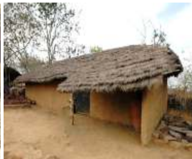
Adobe walls with thatch gabled roof - Uttar Pradesh
