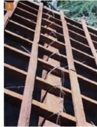
Connection of purlins & rafters, and beam & rafters.
