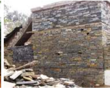
Ashlar Stone Walls with country tiles hipped roof- Chattisgarh
