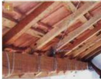
Connection of purlins & rafters, and beam & rafters.
