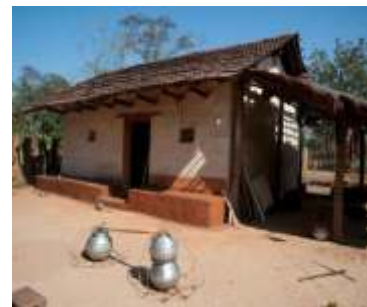
Wattle and daub walls with Mangalore tiles gabled roof - Odisha
