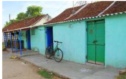
Burnt Brick walls with country tiles gabled roof- West Bengal
