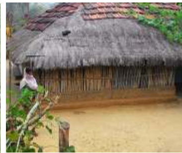
Wattle and daub walls with thatch/ filed hipped roof - Jharkhand
