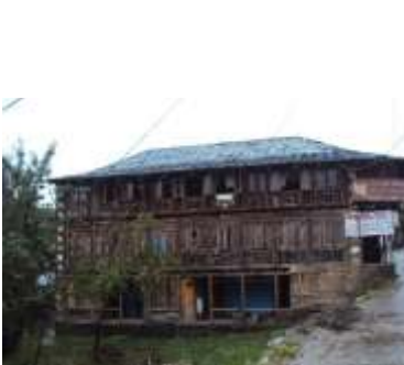
Timber walls with slate stone hipped roof- Himachal Pradesh
