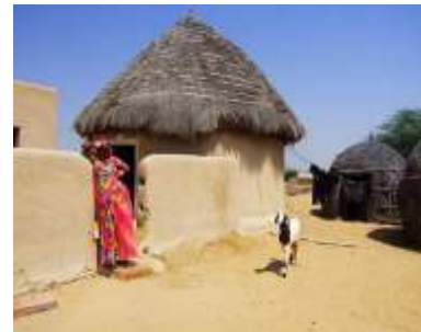
Cob walls with thatch roof over circular plan - Gujarat
