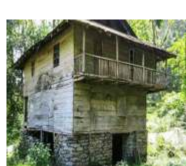
Timber walls with CGI sheet hipped roof- Sikkim
