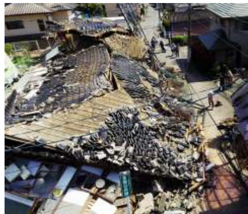
Damage to heavy roof due to earthquake
