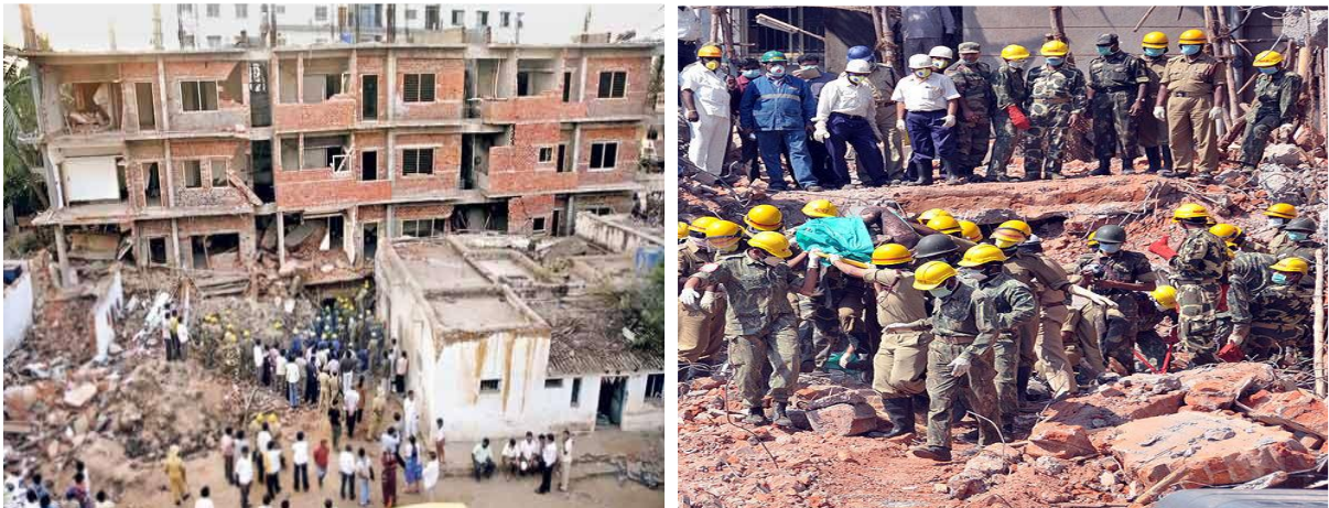
Building Collapse in Ballari, Collected from Hindu News Paper
