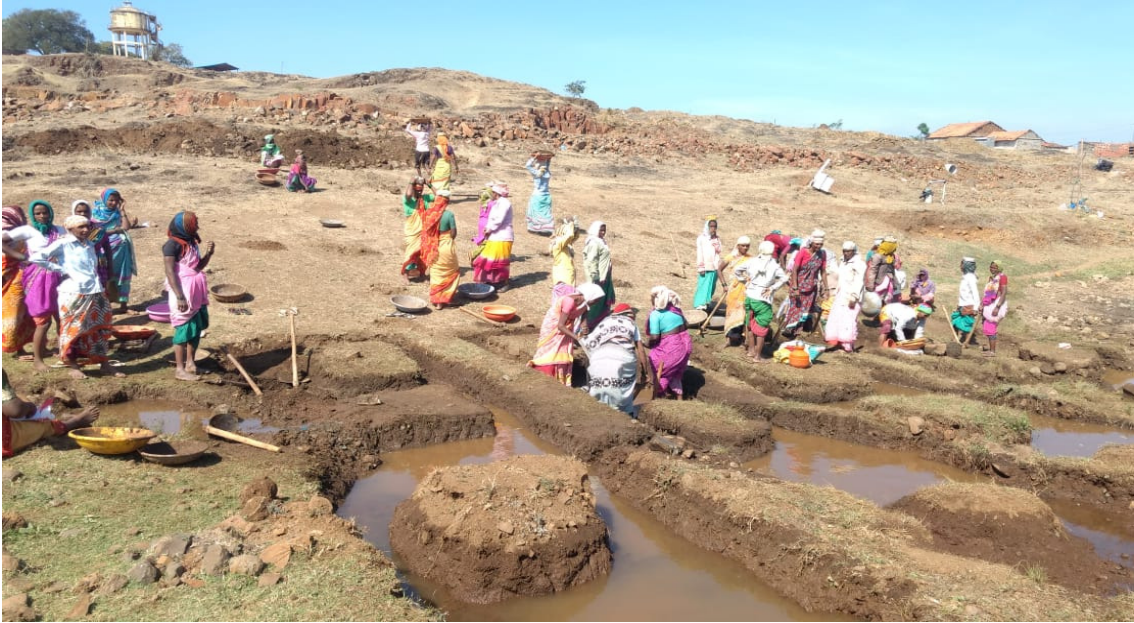
Tank Desilting Work Wadral GP, Chikkodi Taluka
