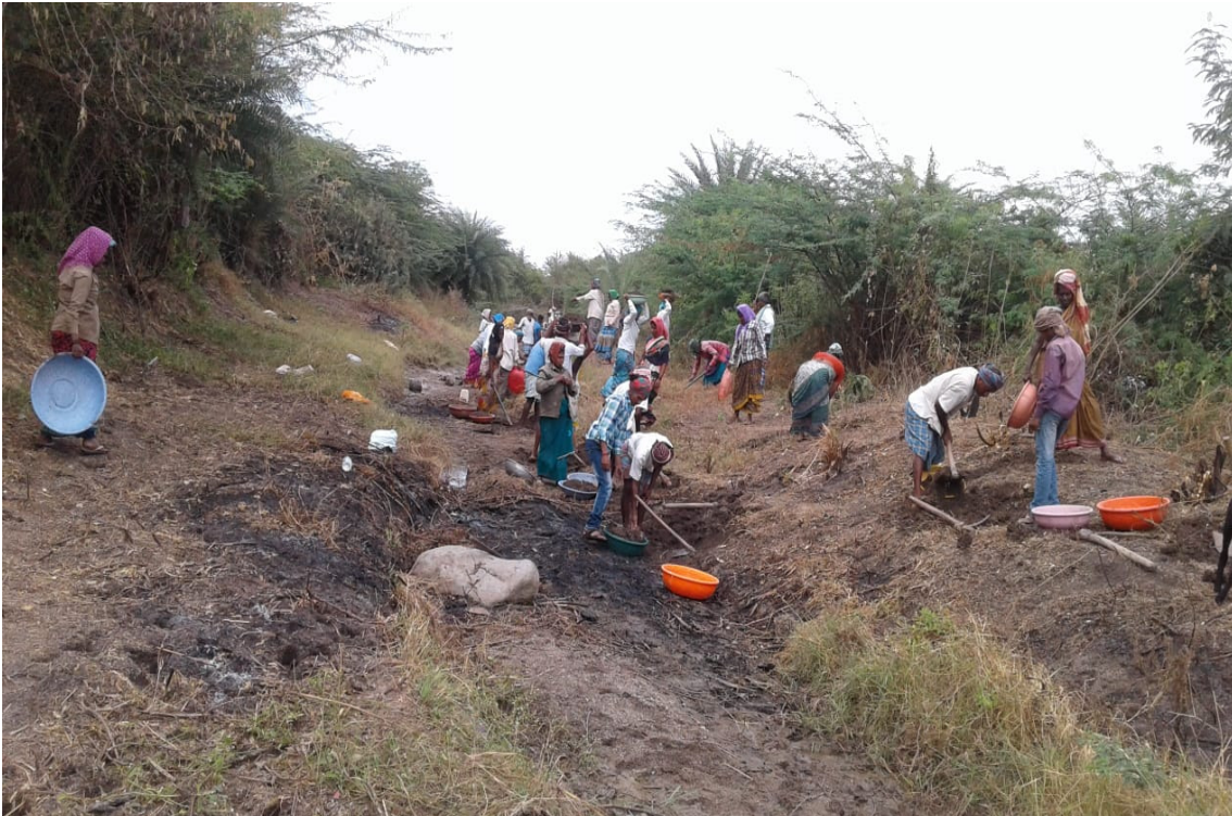
Nala Desilting Work Asundi GP, Savadatti Taluka
