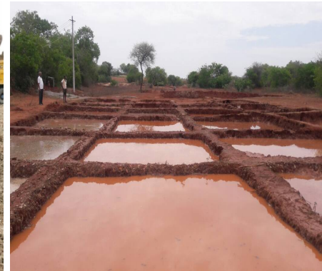
Water Filled After Desiltation
