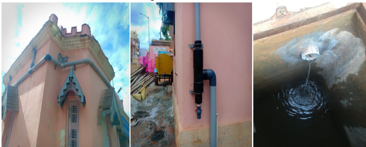
Roof Top Rain Water Harvesting
