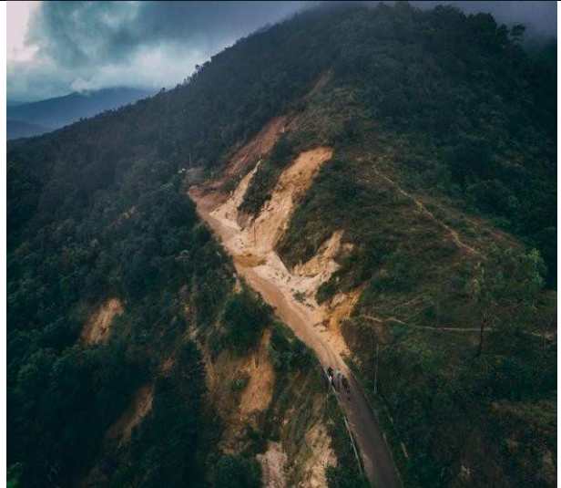
Bird view of Multiple Debris slides occurred along Hirebail-Hemmakki road at Malleshwaragudda
