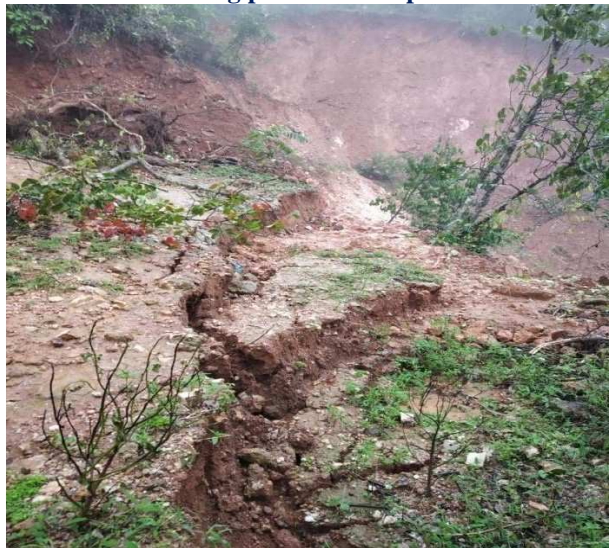
Large crack & subsidence observed near crown
