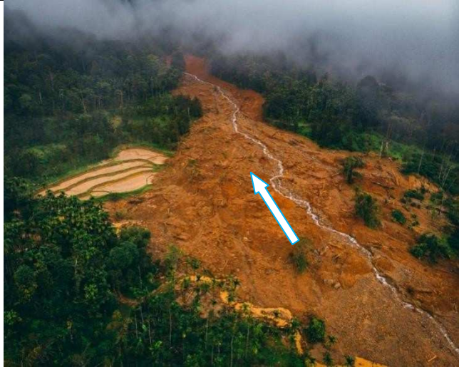
Rapid flow of debris at downhill slide, destroyed the plantation
