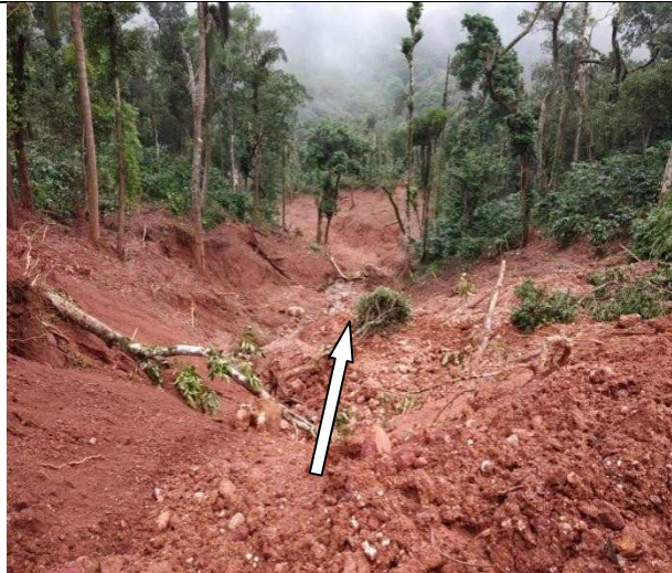
Debris slides consuming part of coffee plantation at downslope
