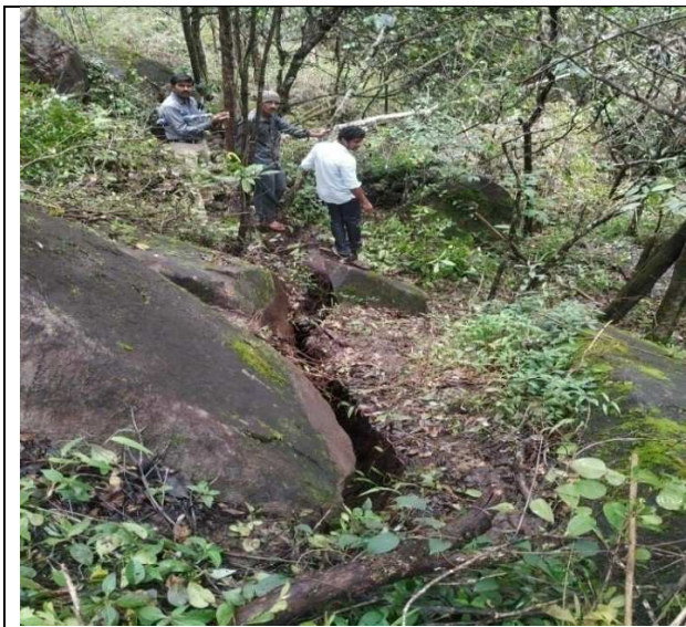
Large size arc shape crack observed on top of the hill
