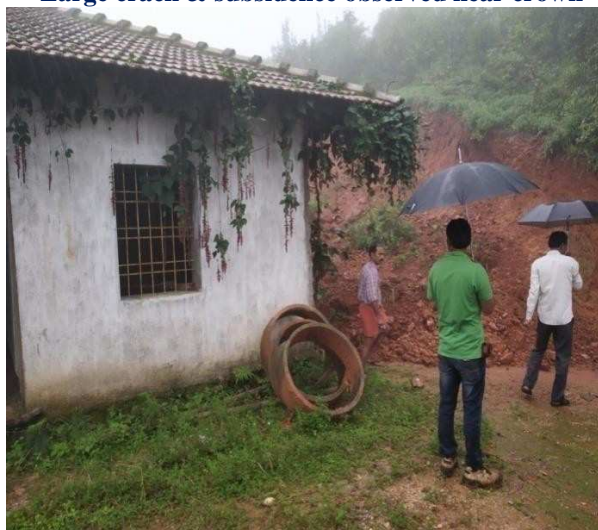
Partly damage house near the crown part of slide
