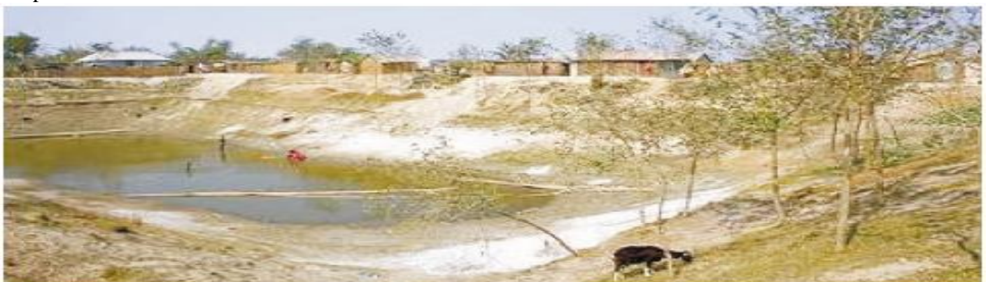
- Khash Dhalai Flood Shelter
