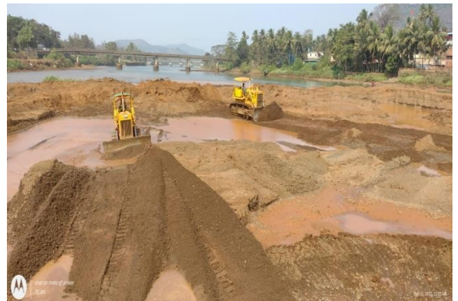
Photo 2 Desilting of silt at Vashiti River
