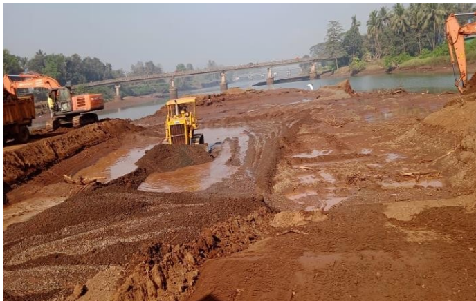
Photo 2 Desilting of silt at Vashiti River
