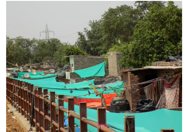
Green nets installed in Kishan Kunj
