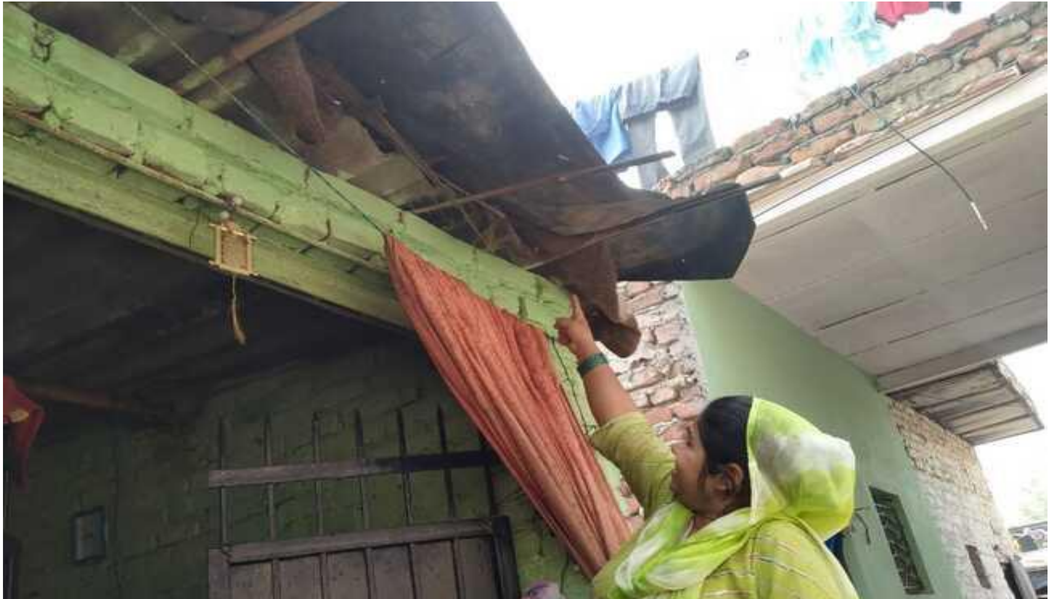
Cool roof intervention , Kishan Kunj, East Delhi
