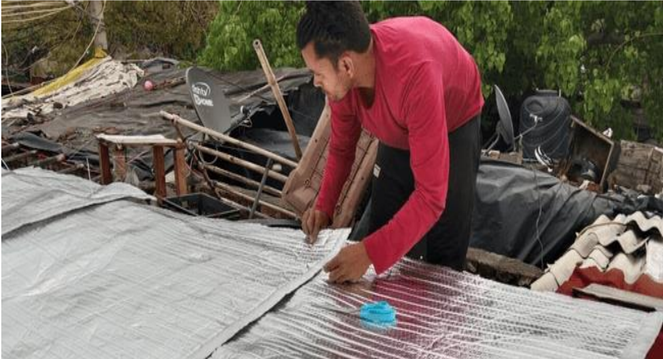
Cool roof intervention , Kishan Kunj, East Delhi
