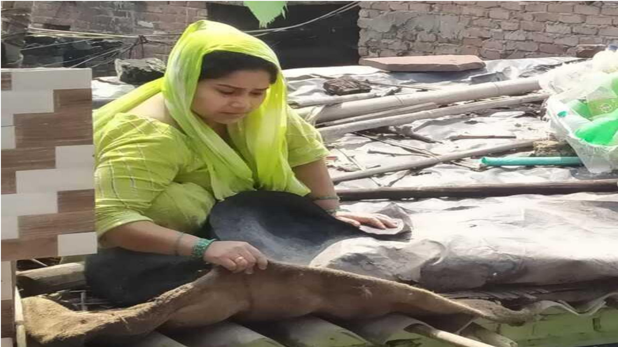
Cool roof intervention , Kishan Kunj, East Delhi
